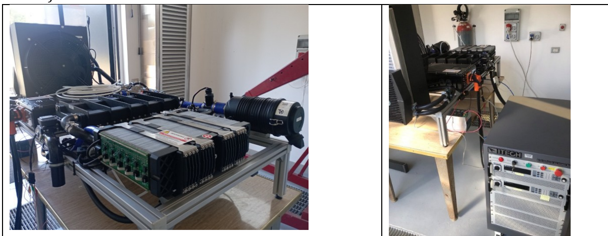
Figure 4. Pictures of the experimental setup showing the fuel cell system (left) and the bidirectional electronic load (right)
