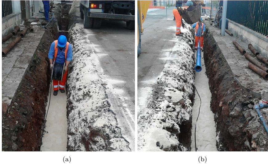
Figure 5: Installation of the two-element cable (a); Installation of the pipe (b).
