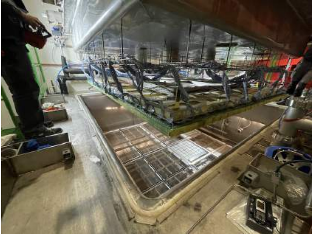
Figure 1.9. The cold box during installation of a CRP. The cathode is visible on the bottom, with an X-ARAPUCA PD installed.
