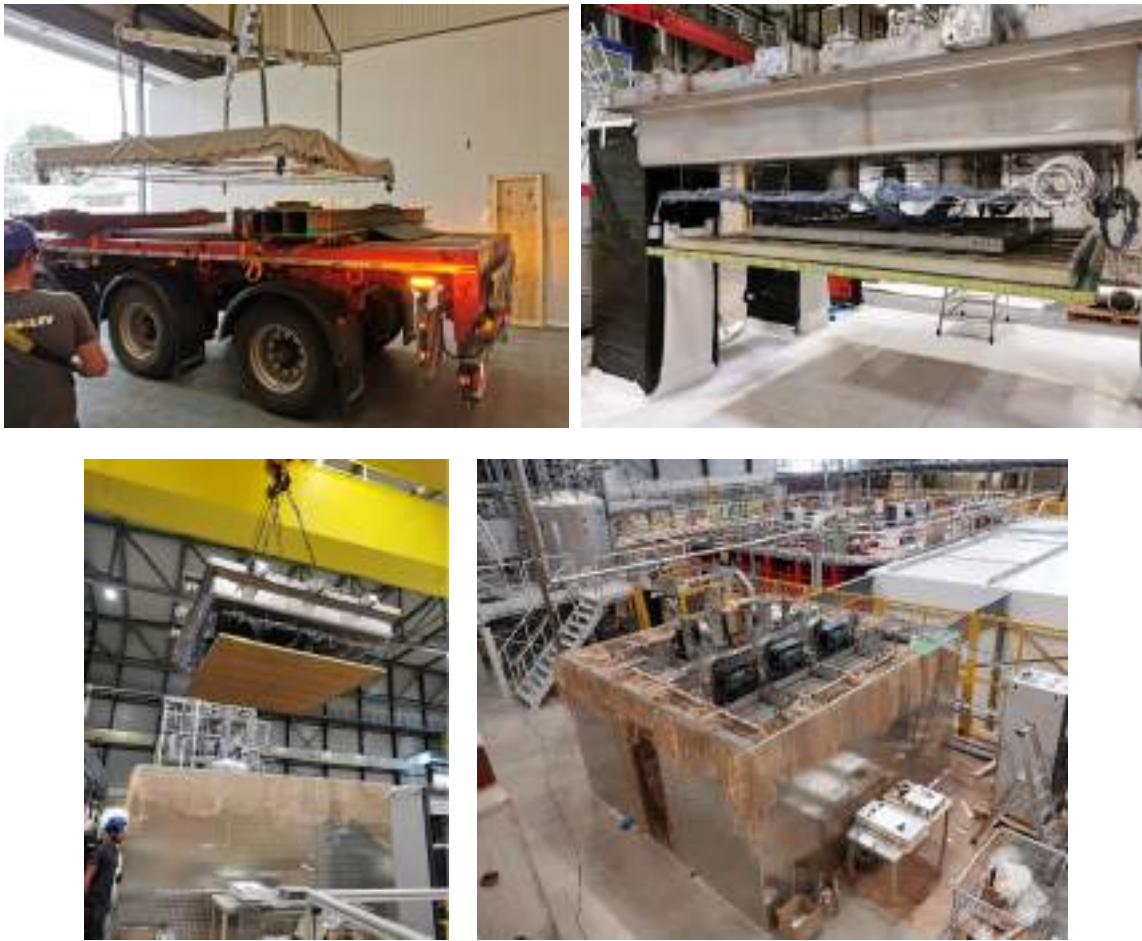
Figure 3.40. Top left: CRP-2 inside the transport box is being loaded to a truck for the transport to EHN1. Top right: at EHN1, CPR-2 is attached to the cold box roof and raised to the final height. Bottom Left: the cold box roof with the attached CRP-2 is on its way to the Faraday cage. Bottom Right: the cold box roof positioned at its final position on the Faraday cage room.
