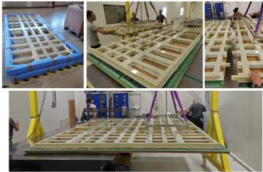
Figure 3.37. Top left: two halves of the composite frame as received from the manufacturer. Top middle: half composites are attached to the anode assembly and they are ready to be connected. Top right: connecting two half units. Bottom: composite frames are connected and assembly is ready for the edge card installation.
