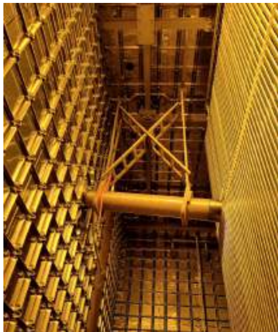
Figure 8.14. Photo of the beam plug realized and installed in the FD1-HD Module 0 .
