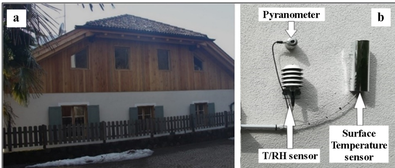
Figure 4. (a) Northeast wall monitored. (b) External sensors installed (Pyranometer, T/RH sensor, Surface temperature sensor).
