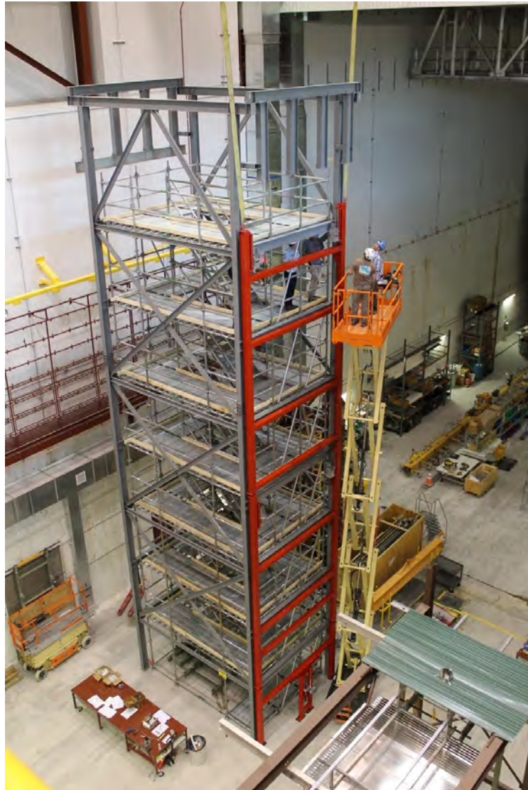
Figure 4.6. Phase 1 APA installation frame (in red) being installed on the APA assembly tower at Ash River. In the foreground is the ProtoDUNE-SP trial assembly structure.
