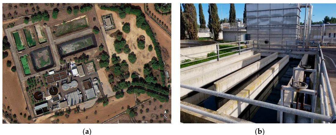
Figure 1. (a) Detailed view of the plant layout highlighting the main treatment units; (b) photograph of the chlorine contact tank, which constitutes the subject of the hydraulics and CFD analyses presented in this study.
